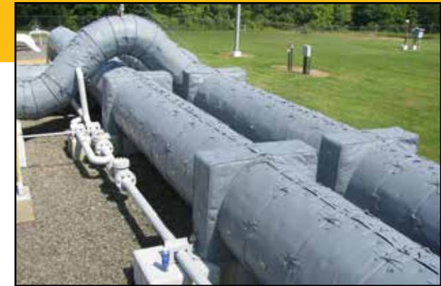
LT450A-TT NATURAL GAS PIPELINE 24" (13 dBA REDUCTION)
