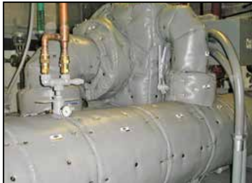
LT250A-VP CENTRIFUGAL LIQUID CHILLER (8 dBA REDUCTION)
