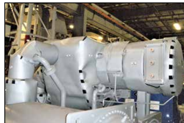
LT250AS CENTRIFUGAL LIQUID CHILLER (6 dBA REDUCTION)
