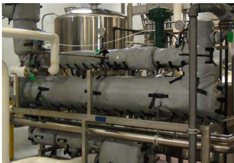
STEAM PASTEURIZING HEAT EXCHANGER PIPING & FITTINGS
